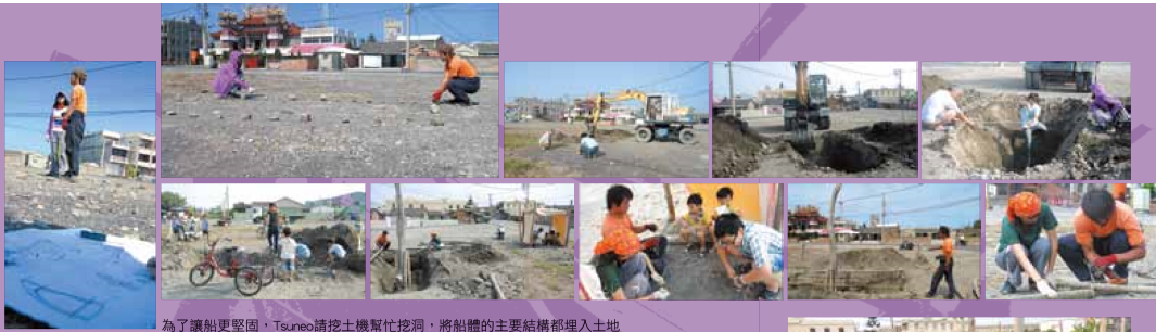
為了讓船更堅固，Tsuneo請挖土機幫忙挖洞，將船體的主要結構都埋入土地。 In order to make the boat as strong as possible, an excavator was asked to dig a hole for putting part of the main structure in the land.
