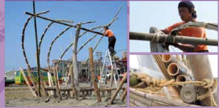
為了避免大風把船吹翻了，Tsuneo將船帆製作成可拆卸的，讓村民可以在颶風天及下雨天幫忙收起船帆。 In order to avoid strong winds blowing away the boat, Tsuneo made the sail removable; then the villagers can help take down the sail before typhoons and rainy days.
